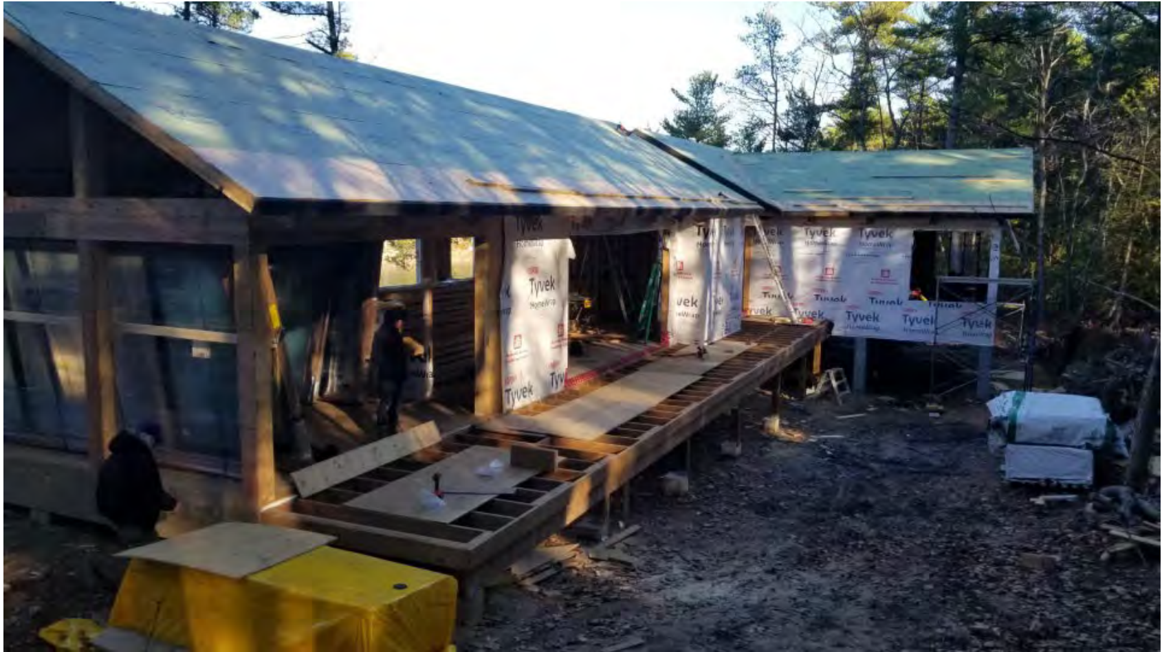
SITE PHOTO TAKEN OCTOBER, 2022
