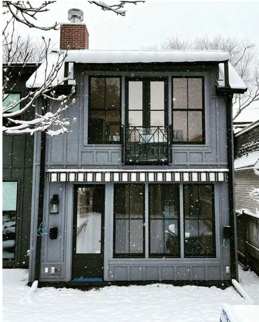
SITE PHOTO OF REAR ADDITION, TAKEN FEBRUARY 2022
